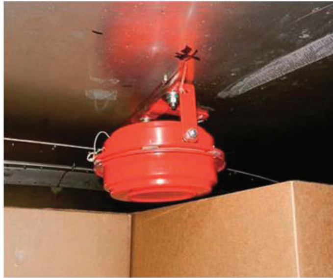
Figure 6.2. In-container fire suppression system
